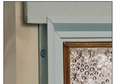
Plasterboard cover trim slots into the channel
